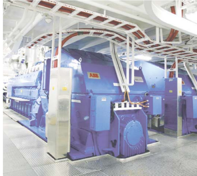
Generator installation on an advanced OSV with electric propulsion
